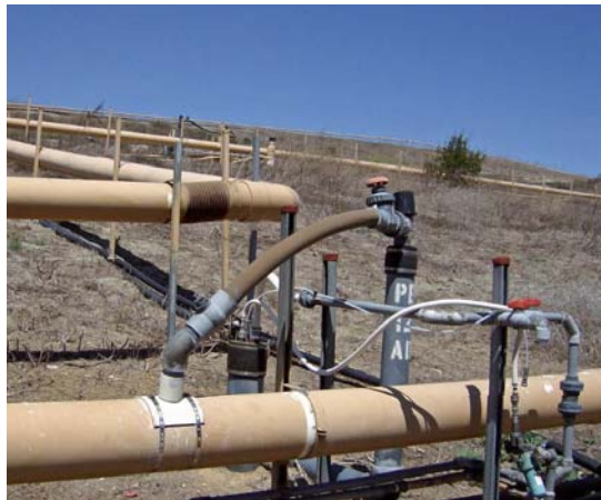
Methane well and gas collection pipes
